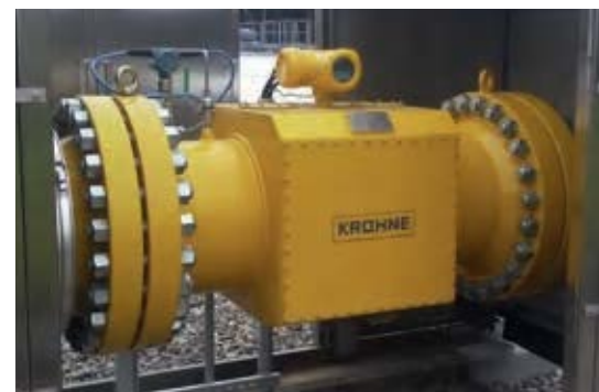
Custody transfer flow measurement for a bidirectional natural gas border metering station
