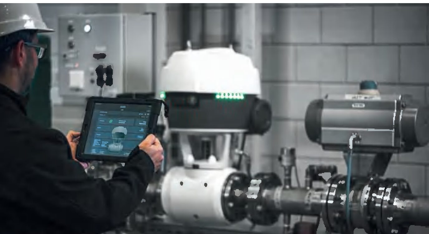
FOCUS-1 DN 80 in a flow control application
