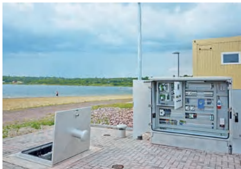
Measurement of disinfectants with remote data communication
